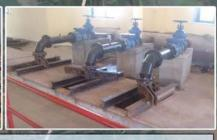
The Jack well is constructed at Veer Dam. The present work is for providing 3 nos x 80 hp Raw Water Pumping machinery (2 w + 1 Stand by) at Jack well along with all allied materials like panel, cables, valves, delivery mains etc and also providing 2 nos. 200 KVA Transformers in the existing substation at jack well at Veer Dam along with all allied material like Do set, AB switch, Disc & pin insulators etc.
